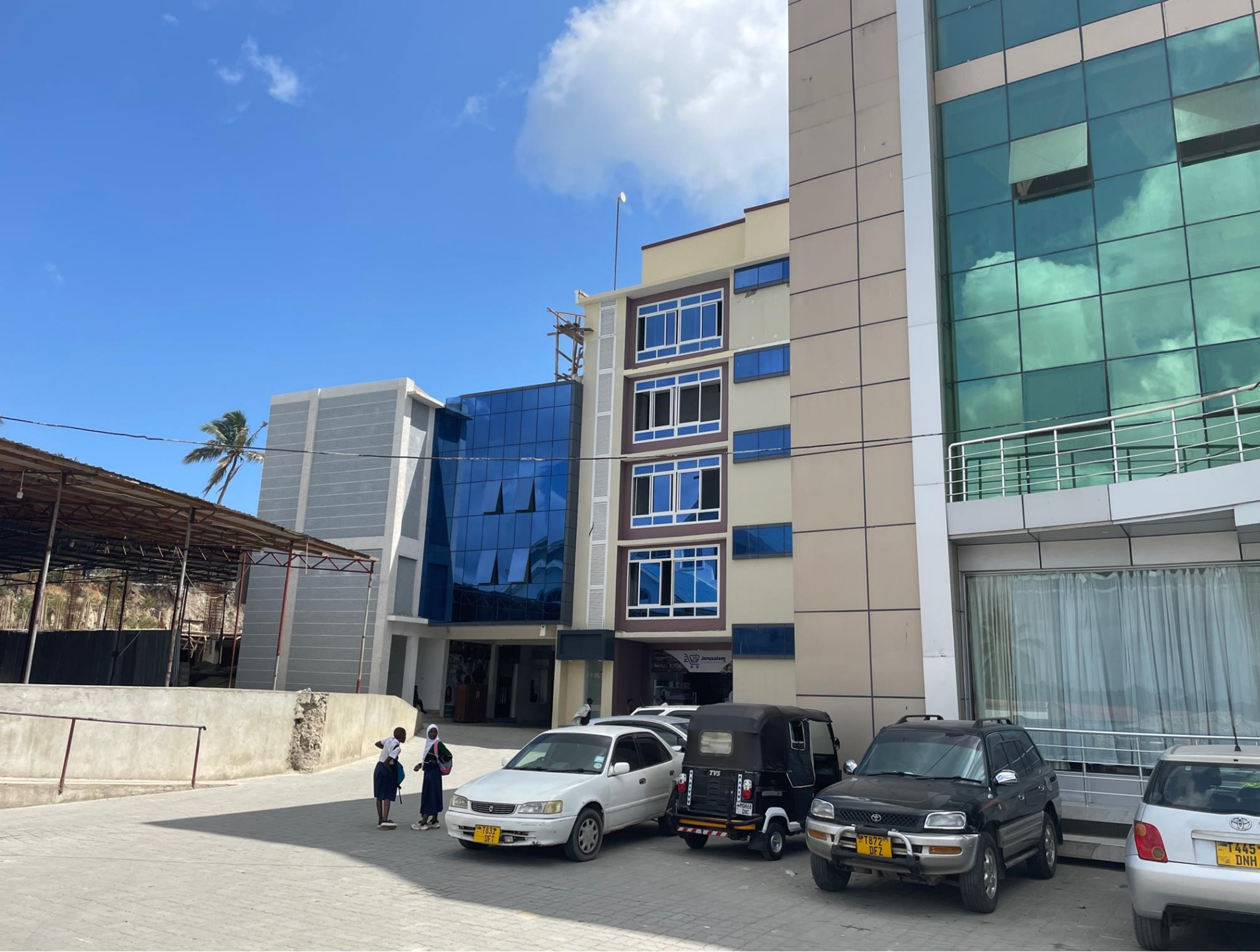
At Kimara, Church, Hospital
